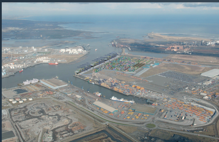
▲ The INEOS plant at Teesport
