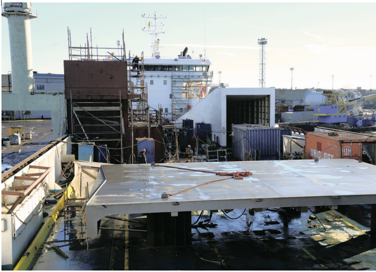
▲ Important: The new side port was already onboard SC Ahtela when TransNytt visited the vessel in early February. The side port itself looks rather “stupid” as it lays on the weather deck, but the extensive equipment needed to operate it makes the side port state-of-the-art.
