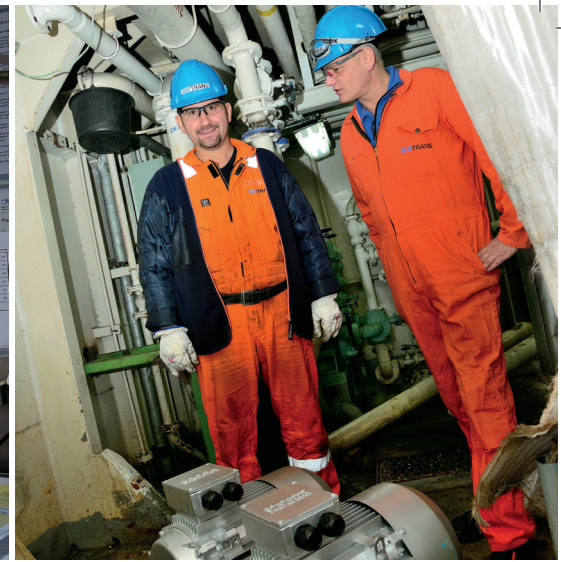
▲ New pumps: Some brand new equipment was brought onboard, such as two pumps for high pressure air, installed by 2nd Engineer Camarasu Nicosur to the left.
